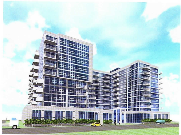
In August, Main Architecture celebrated 40 years as a design and architecture firm. Located in downtown Chicago on Wabash Avenue, Main has designed award-winning structures, which include Paramount Lofts and Motor Row Condominiums.
