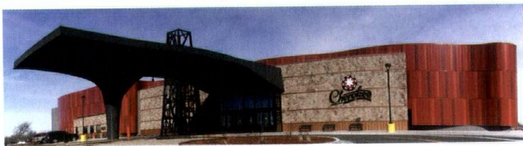
Cherokee Casino Ramona in Ramona, OK Owner: Cherokee Nation Entertainment, Architect: Selser Schaefer Architects, Contractor: RMZ Builders Installer: Abbco Roofing; Profiles: Perforated Flush Panel, Flush Panel, PAC Precision Series HWP, 7.2 Panel, 7/8" Corrugated, Flat Sheet; Colors: Colonial Red, custom Bright Red, Copper Penny, Slate Gray
