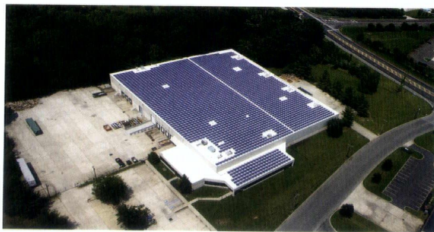
Birds-eye view of McGrory's 108,000 square foot solar powered facility, located in Paulsboro, New Jersey
