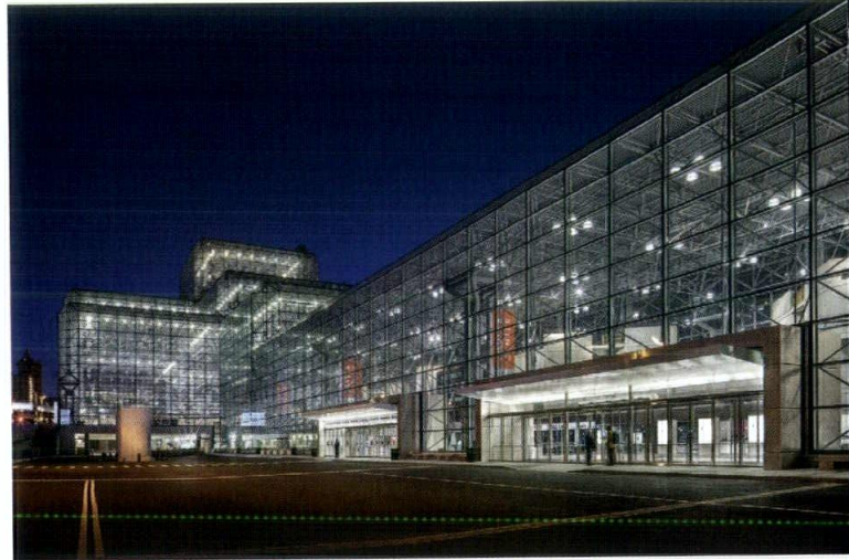
Photo by Esto Photographics Inc
