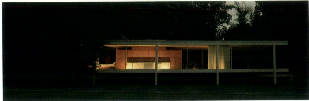
Floodwaters from the Fox River have reached above the floor of Mies' modernist masterpiece at least once every 15 years on average. Studies confirm the frequency of flooding will increase.
