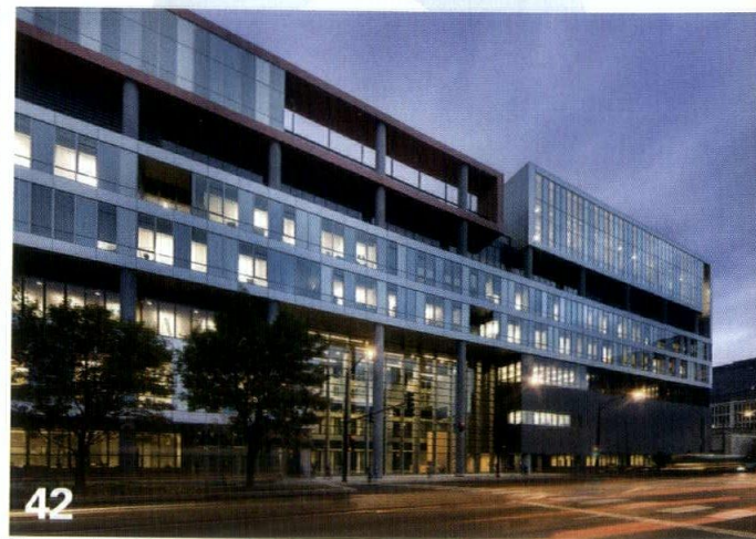
Photo by James Steinkamp, Steinkamp Photography
