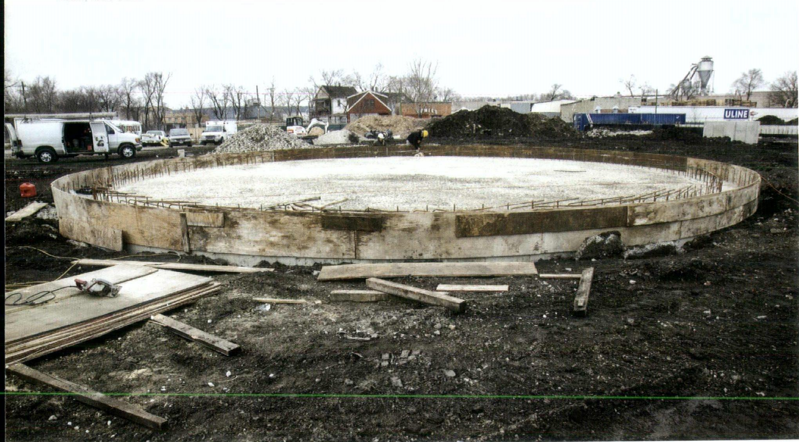
The first of its kind in Chicago, the waste digester will take in 30 tons of food waste from restaurants and The Plant's resident businesses each day, and will put out 400 kilowatt hours of power.
