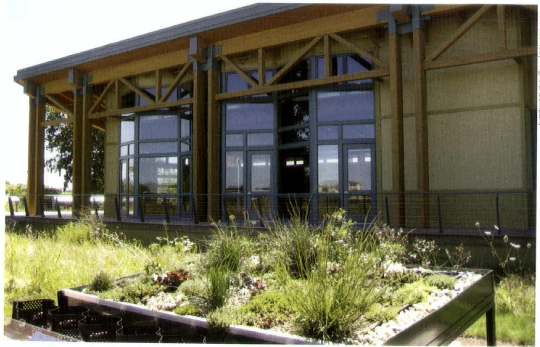
The Evelyn Pease Tyner Interpretive Center in Glenview is an early LEED-NC Platinum building. The roof has solar panels at one end and vegetation at the other, which controls stormwater runoff as part of a low impact development strategy.
