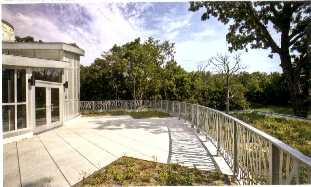
Hidden Oaks Nature Center in Bolingbrook is a LEED-NC v2.2 Platinum project that used LID strategies. The native plants in the green roof require no irrigation.
