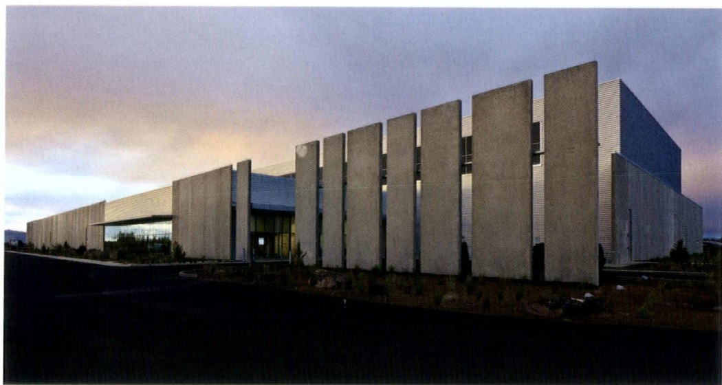
Top: Server room in Prineville Data Center. The open pathway on the right is the “cold aisle.” Bottom: Pre-cast concrete walls not only provide security, but also house courtyards, bringing light into the building, and provide outdoor areas for employees.
