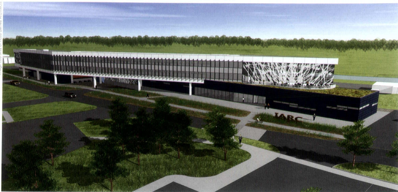
Among Ross Barney Architects' public sector projects is the 42,000-square-foot Illinois Accelerator Research Center at Fermilab in Batavia.
