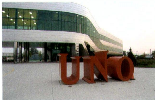
Viewed from a distance, the raised section of the building gives it the appearance of taking flight, but it also functions as a weather-protected outdoor space (top). UNO is putting its imprint on neighborhoods (bottom).
