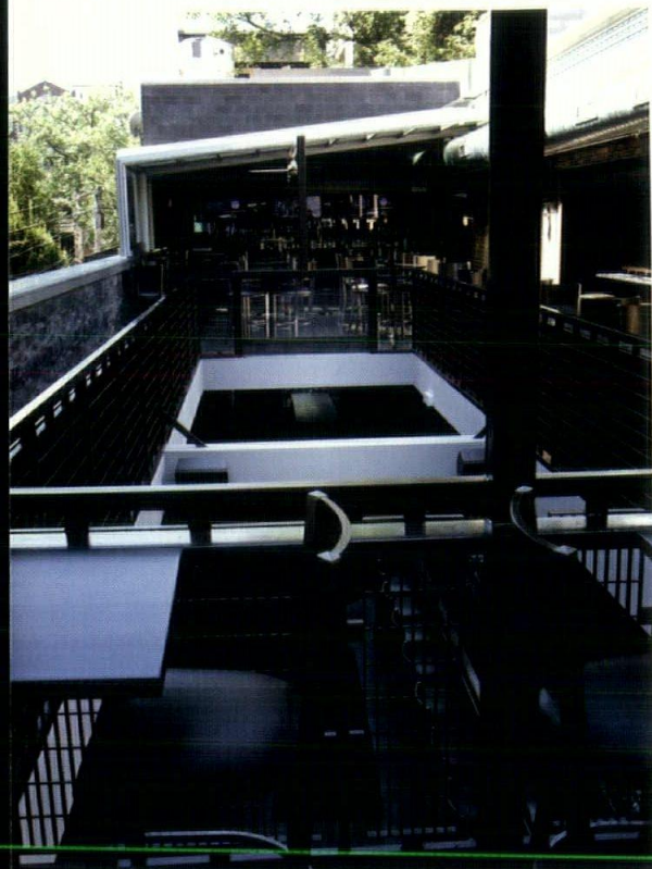
Photo courtesy of the firm
