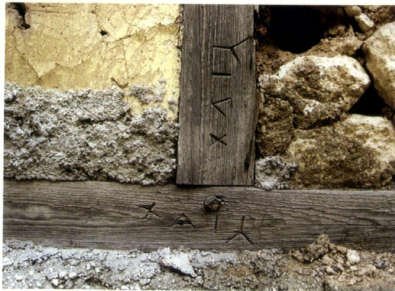
Haiti's Gingerbread houses use both braced-frame construction (timbers secured with wooden pegs, also called treenails) and colombage, or pan de bois , construction (masonry infill wall panels made of bricks or stones laid in mortar). The Roman numerals are carpenter's marks. A third construction type—masonry bearing walls—is also used.
