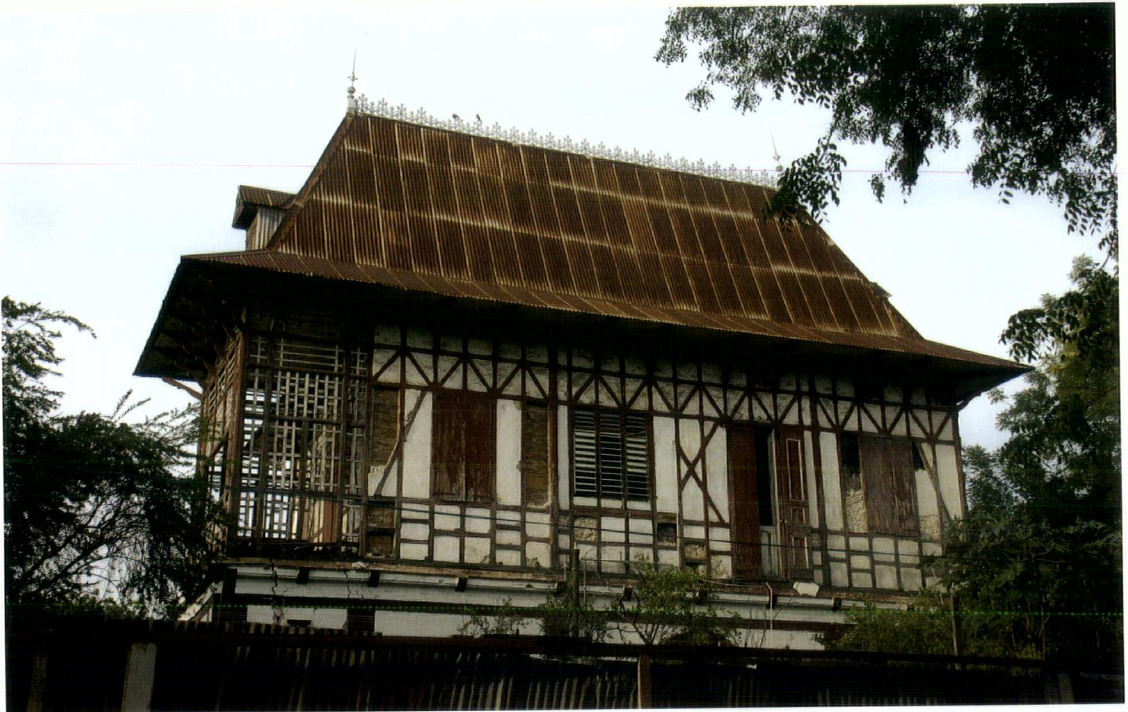
One of the 200 houses in Haiti's Gingerbread district. The metal roof and its spire are typical of Haiti's Gingerbread houses. Panels of stone and mortar were knocked loose by the earthquake.
