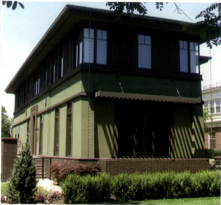
(1) Deep eaves were an aesthetic choice for a home by Paul Florian, but they also provide some weather protection for less-expensive exterior materials.
