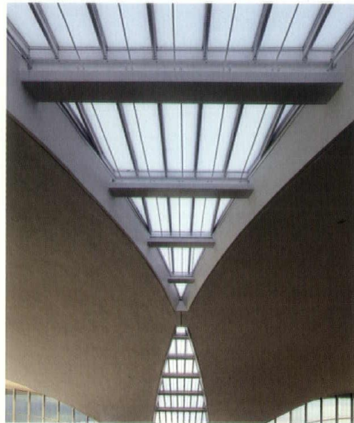
Restored skylights at Lambert-St. Louis International Airport
