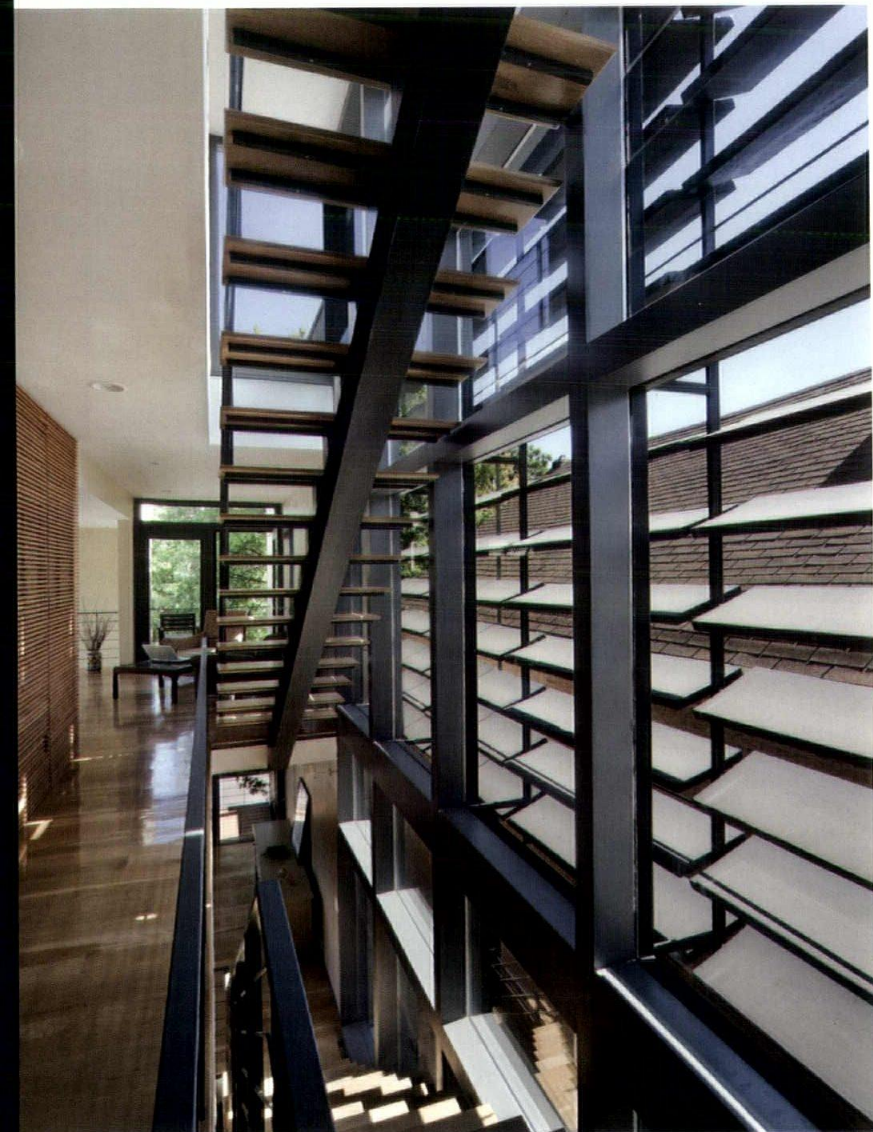
A minimalist staircase rises like a spine beside the home's mostly glass south wall. Hand-operated louvers made of 2 x 12 pressure-treated lumber control sun exposure and the view of the close-set neighbor.
