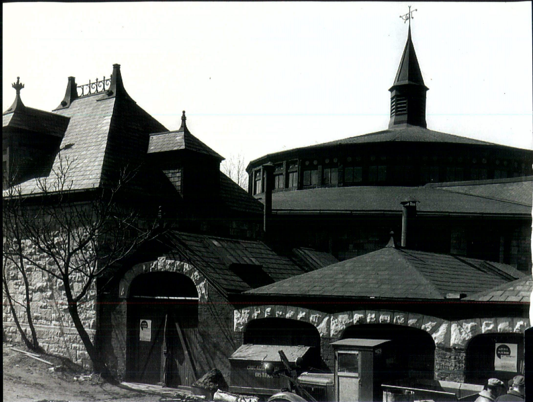
The single existing photograph that guides the Roundhouse Project, restoration of a former horse barn designed by Daniel H. Burnham
