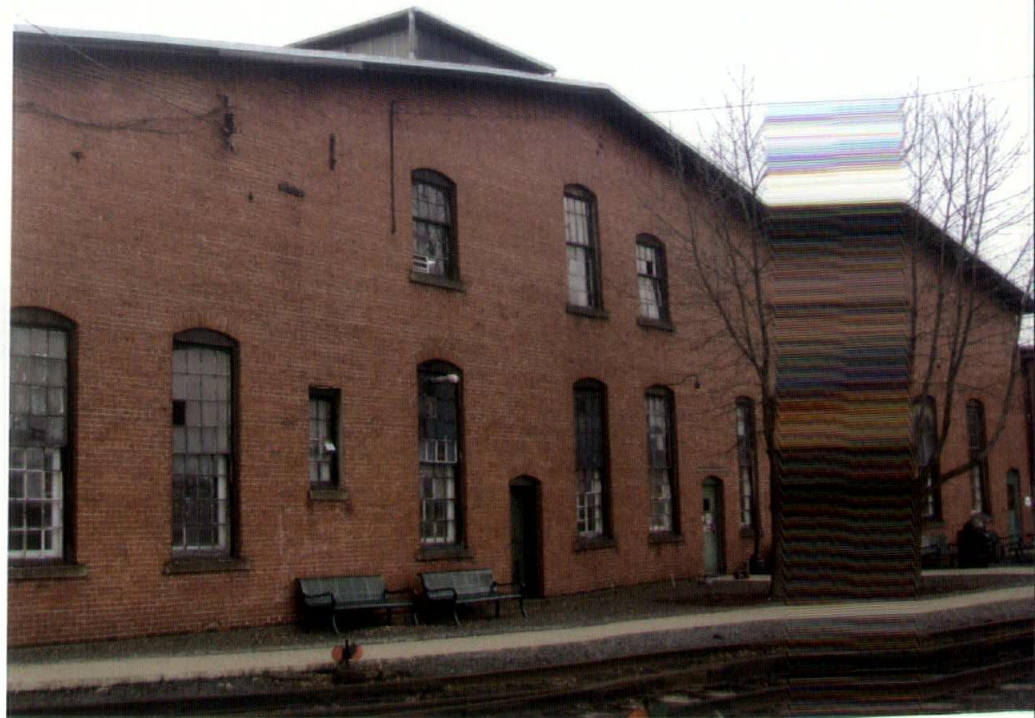
BauerLatoza designed the exterior rehabilitation program for Steamtown's 1865 Locomotive Shop, a railroad equipment repair facility listed on the National Register of Historic Places.
