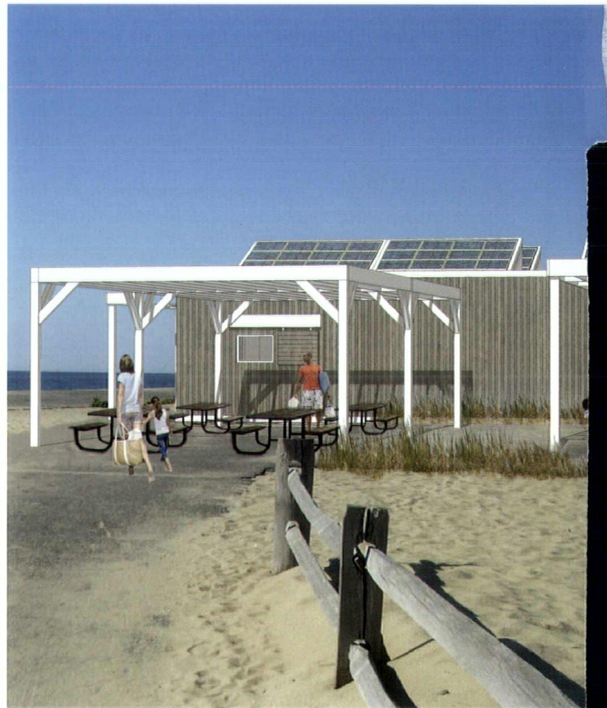
Modular and portable, new utility buildings at Cape Cod National Seashore can be moved to higher ground as the shore erodes.
