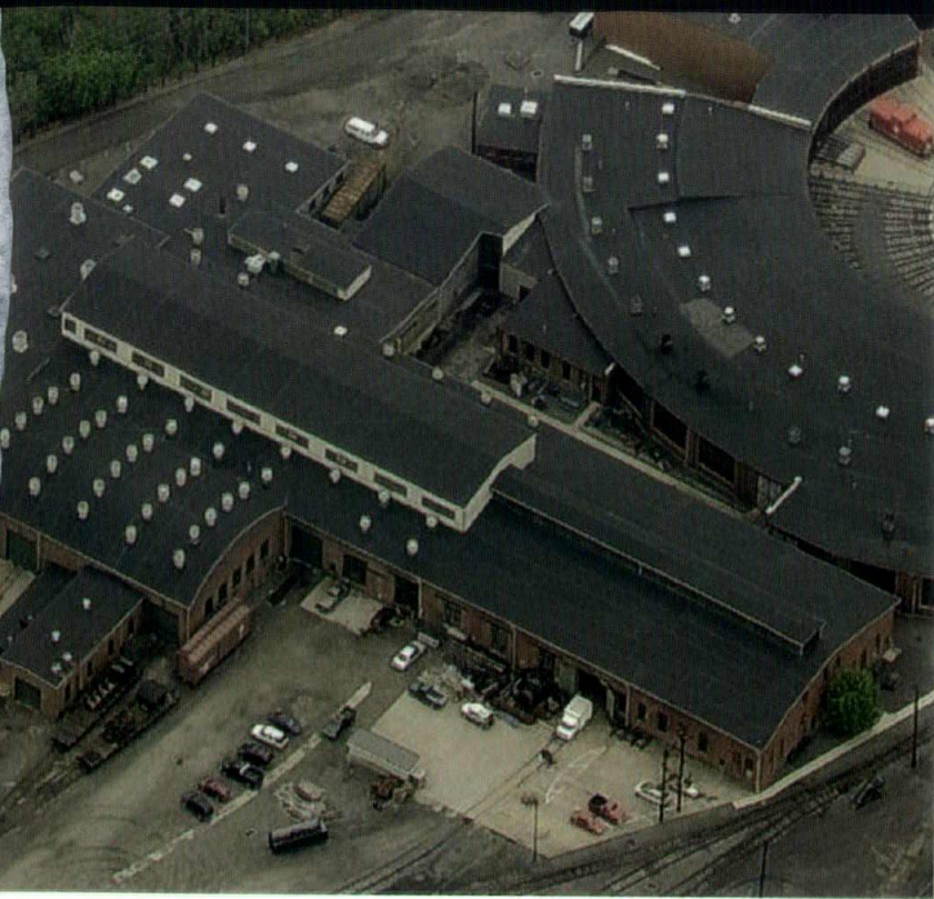
Steamtown's Locomotive Shop will be outfitted with 81,117 square feet of new rubber roofing membrane and 125 new energy-efficient storm windows.
