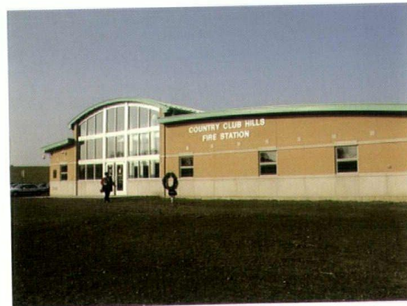
Country Club Hills Fire Station
