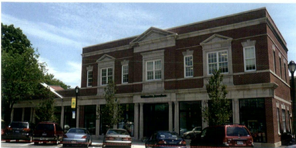
North Shore Community Bank, Wilmette
