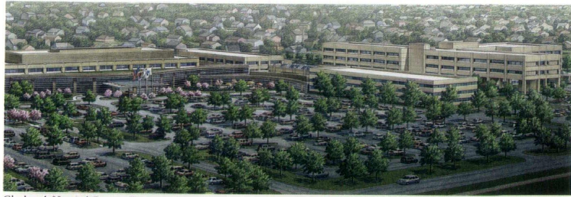
Glenbrook Hospital Campus Expansion
