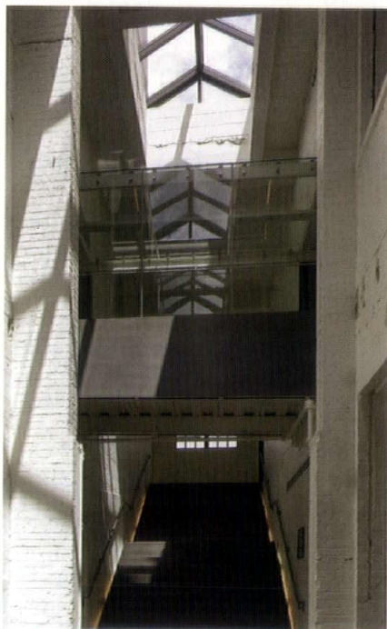
The steel-and-glass stair and bridge connect the original structure to a 1930 annex.
