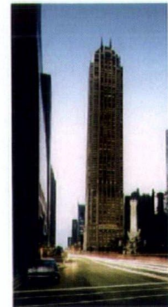
Park Tower Lucien LaGrange
