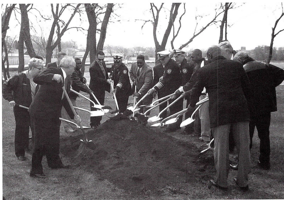
Photo courtesy of the firm
