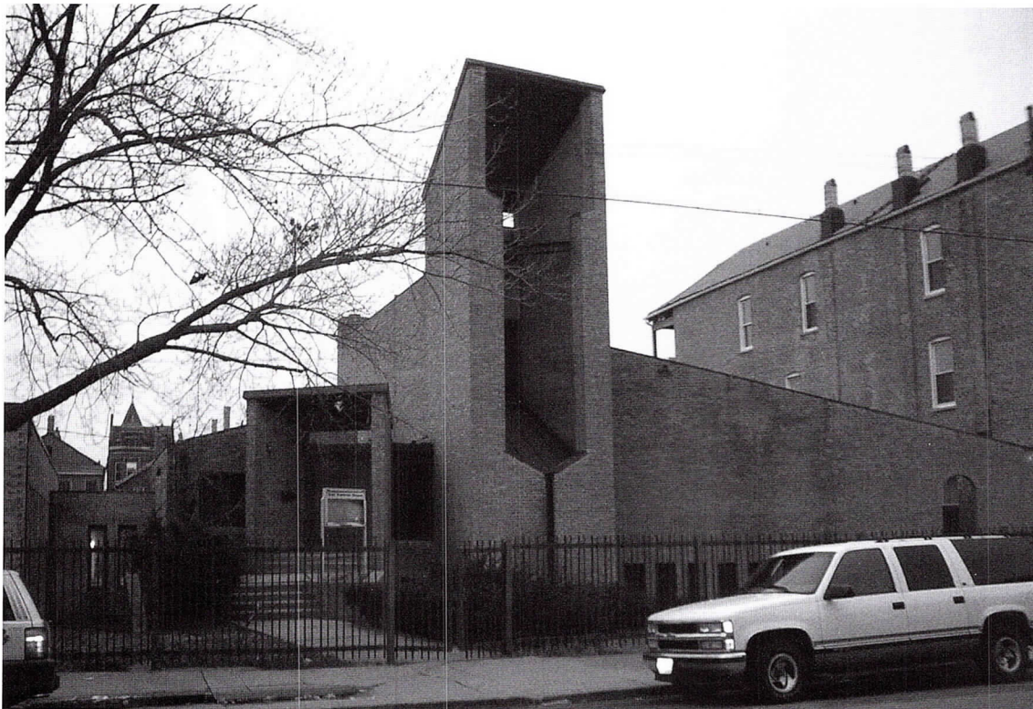
Built of common brick, the charm of Emmanuel Presbyterian is most notable in the use of sunlight inside the worship space. In most of his Chicago churches, Dart used light to maximum dramatic effect. Here, to quote the AIA Guide to Chicago , Dart "made morning light the most powerful architectural element, casting it across the angled chancel wall to create a sense of shelter and spirituality."
