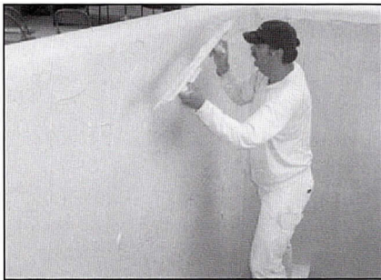
Conventional and Veneer Plaster
