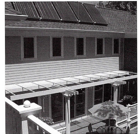
NATHAN KIPNIS ARCHITECTS, INC., ILLINOIS
