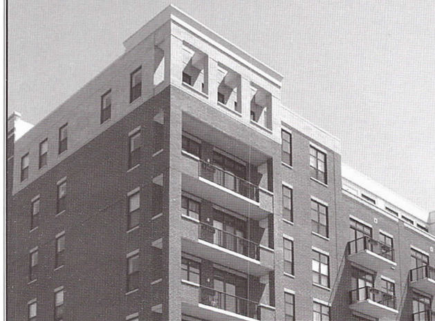
University Village - Midrise Lofts - Total Precast Structural Frame - Chicago, IL
