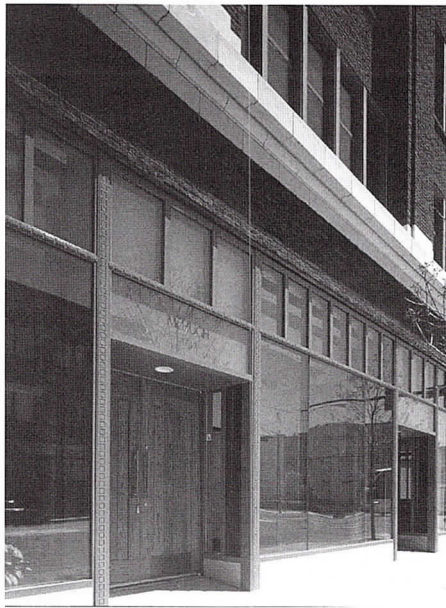
DeStefano and Partners only had one vintage photo to use for recreating the historic storefront for McHugh's new headquarters. The interior of the landmark Maxwell-Briscoe building was gutted.
