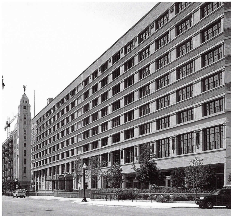
A designated landmark, Gensler worked closely with city officials to keep the 600 W. Chicago Ave. façade historically accurate. White paint was removed from the red brick.
