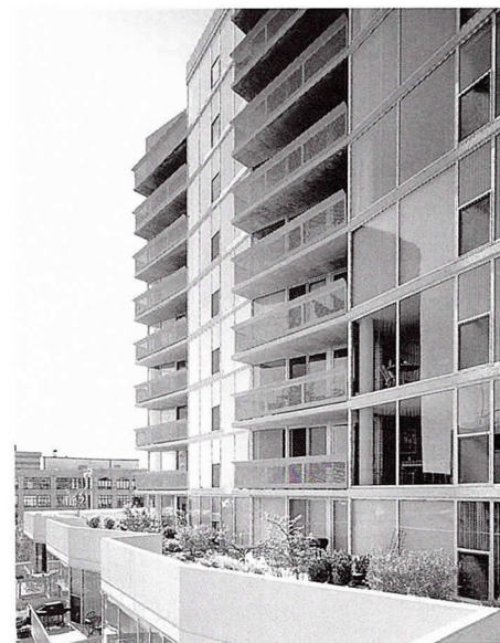
The Towers in Evanston by David Hovey, FAIA of Optima
