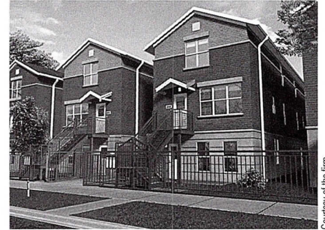
This three-flat in Rockwell Gardens by Piekarz Associates has an accessible ground-floor unit.
