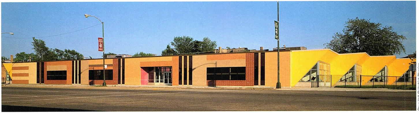
Steve Hall © Hedrich Blessing
