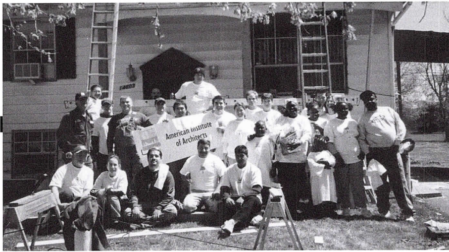
AIA Chicago members repair a Dixmoor house on National Rebuilding Day.
