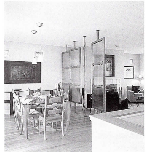
Panels in the Kurtz Residence pivot to provide varying degrees of openness between living and dining areas.
