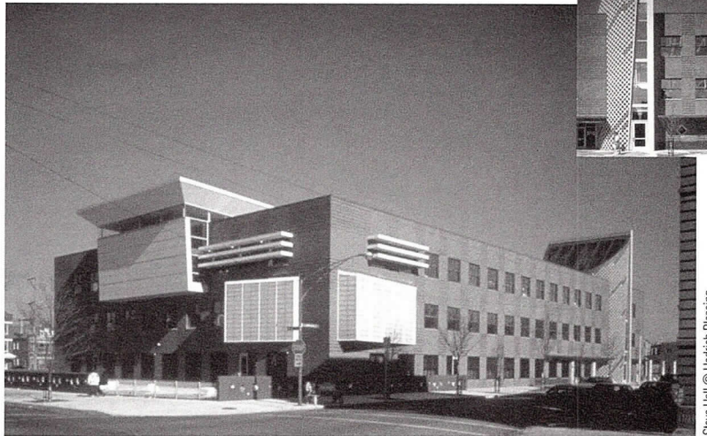
Steve Hall © Hedrich Blessing
