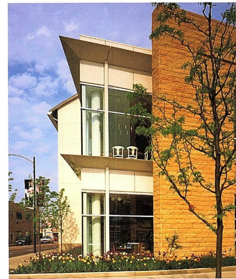
Photo: Jeff @ Hedrich Blessing
