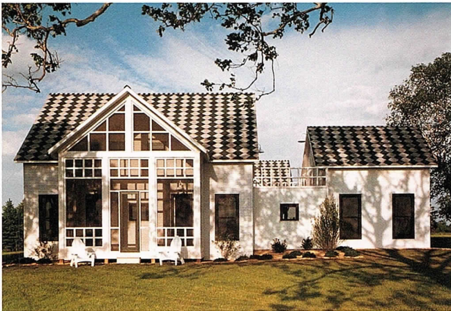
Steve Hall © Hedrich Blessing
