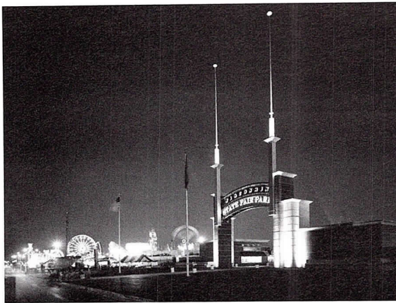
The new main gate of the Wisconsin State Fair by RTKL Associates.
