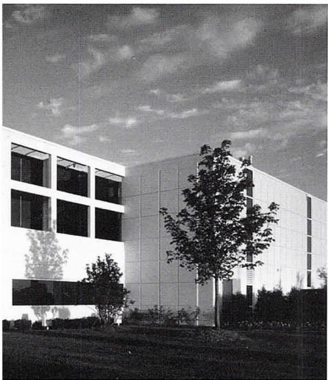
At Systems Research Inc. by RADA Architects, the HVAC units are concealed within the walls of the second floor.
