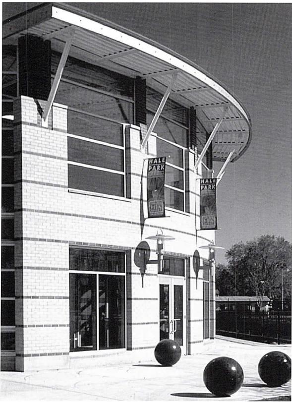
Hale Park Gymnasium 6258 W. 62nd St., Chicago Schroeder Murchie Laya Associates Ltd.
