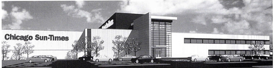
Chicago Sun-Times Production Facility 2800 S. Ashland Ave., Chicago McClier
