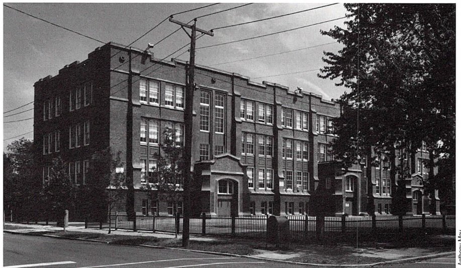
The newly renovated George M. Pullman Elementary School.
