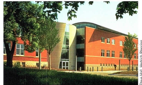
Steve Hall, Hedrich Blessing
