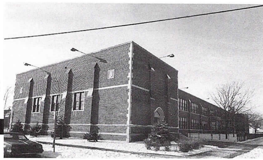
Completed in 1926, the Jonathan Y. Scammon School (far left) at 4201 W. Henderson Ave. was designed by John Christenson. Over the years, renovations have stripped the school of its original architectural ornamentation and windows (left).
