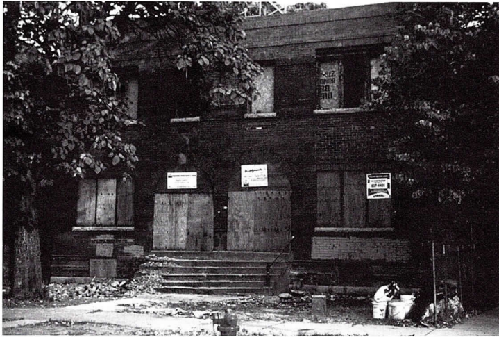
3300 W. LeMoyné St. before rehabilitation began. The project will be completed this spring.
