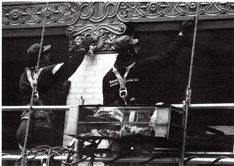
Terra Cotta Cleaning—The Rookery Lightwell
