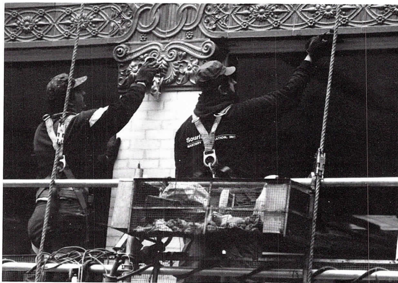
Terra Cotta Cleaning—The Rookery Lightwell
