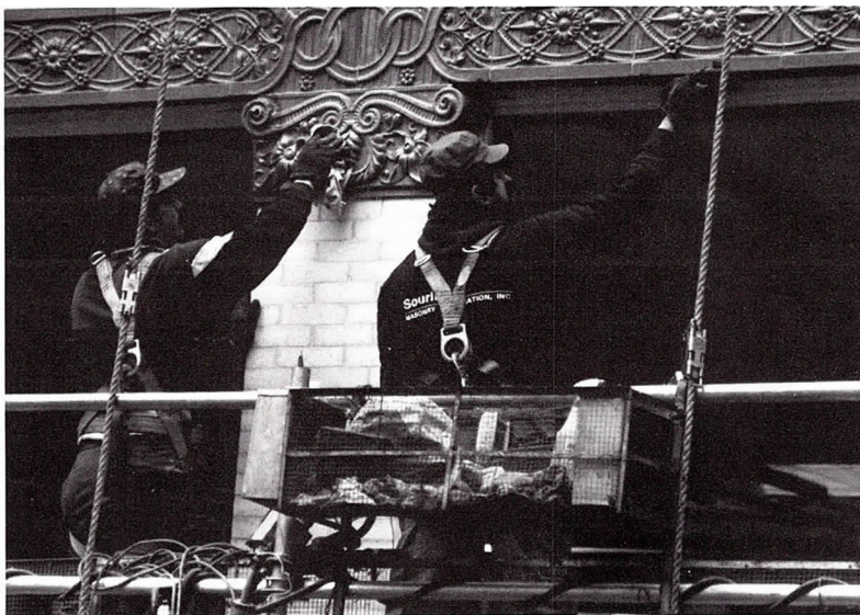
Terra Cotta Cleaning—The Rookery Lightwell
