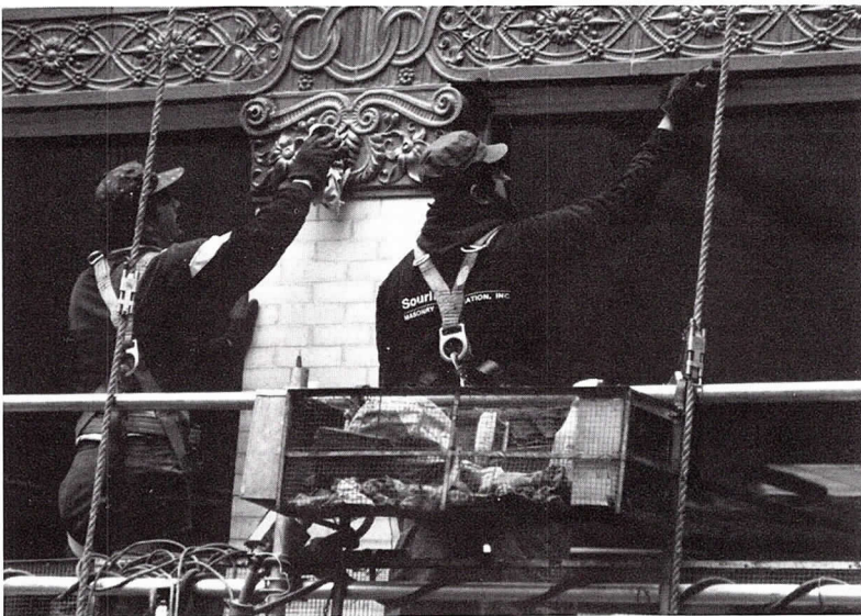
Terra Cotta Cleaning—The Rookery Lightwell
