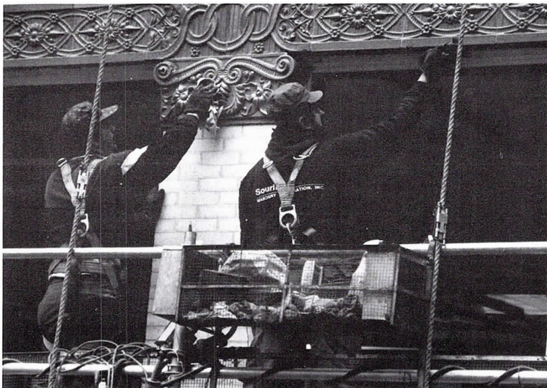
Terra Cotta Cleaning—The Rookery Lightwell
