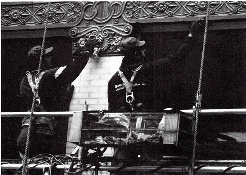
Terra Cotta Cleaning—The Rookery Lightwell
