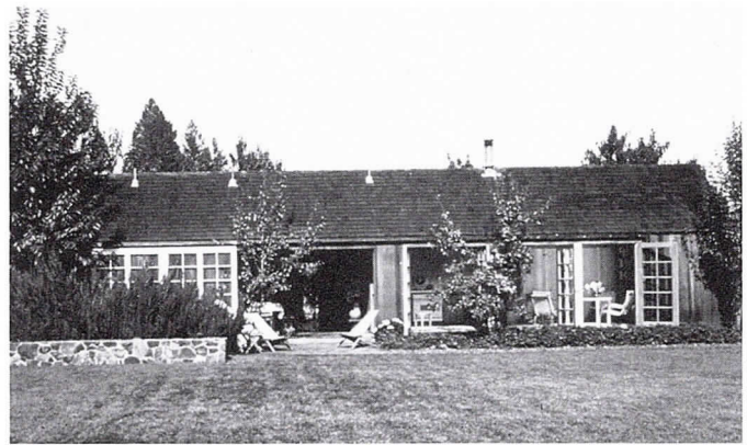
Teviot Springs Vineyard by William Turnbull Associates. Photo by Mark Darley/ESTO.
