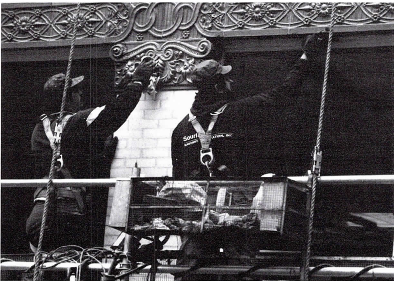
Terra Cotta Cleaning—The Rookery Lightwell
