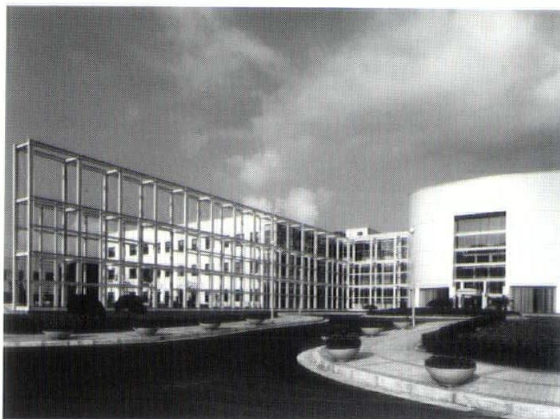
Sam Yang Research Complex Taejon, South Korea Perkins & Will Photographer: Youngchae Park
