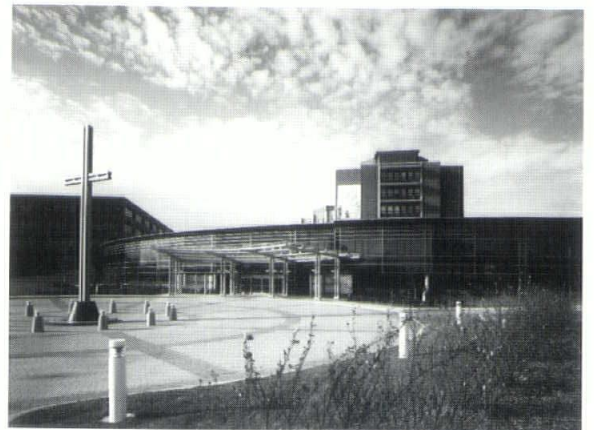
Alexian Brothers Medical Center, East Pavilion Elk Grove Village, Illinois Loebl Schlossman and Hackl, Inc. Photographer: Steinkamp/Ballogg, James Steinkamp
