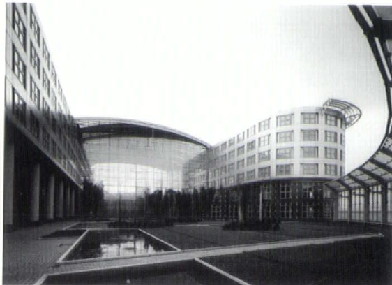
Hyatt Regency Roissy Roissy, France Murphy/Jahn, Inc. Photographer: Images Publishing, Tim Griffith
