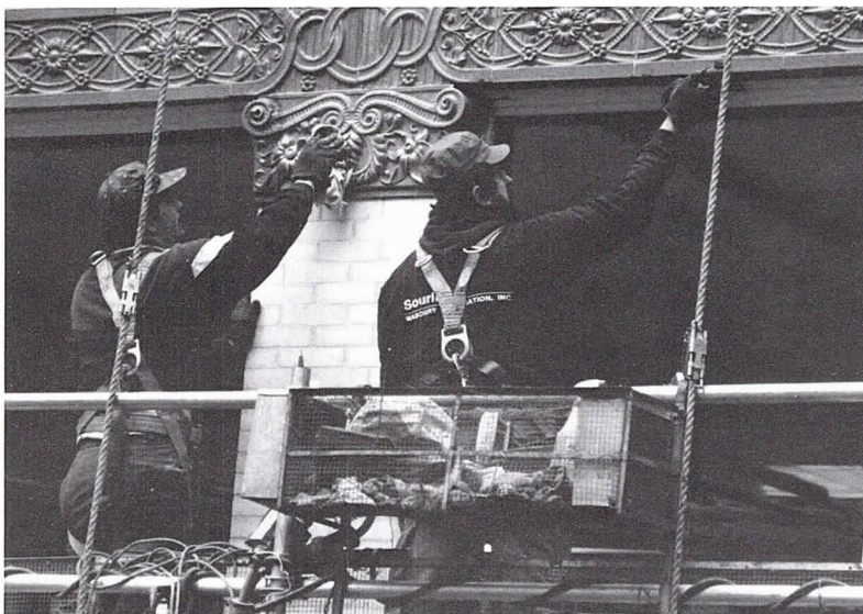
Terra Cotta Cleaning—The Rookery Lightwell
