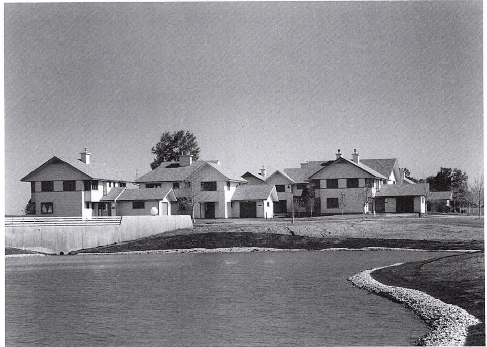
SOS Children's Village in Lockport, Illinois resulted from the efforts of three Chicago architects. Photo by Howard N. Kaplan.
