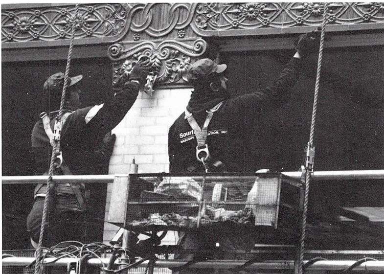
Terra Cotta Cleaning—The Rookery Lightwell
