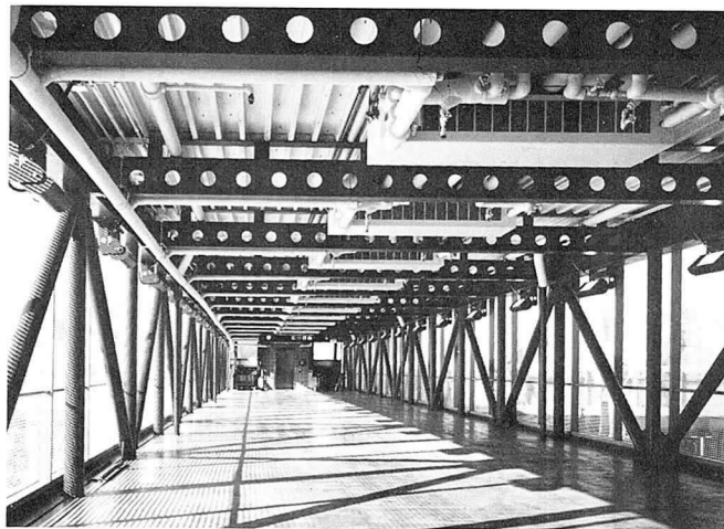
Pedestrian Bridge at O'Hare International Airport, Teng & Associates, engineers, and Ross Barney + Jankowski, design architects.
