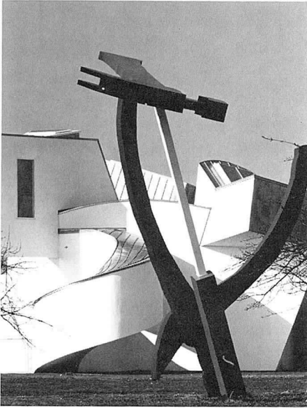
Vitra International Furniture Manufacturing Facility & Design Museum, Weil am Rhine, Germany, one of 10 projects to receive 1992 AIA Honor Award. Frank O. Gehry & Associates. Photo: Richard Bryant
